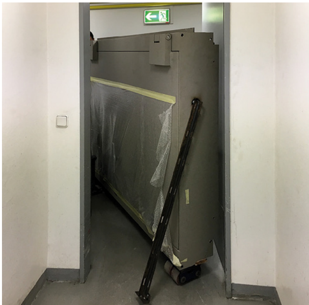
Transport of the vault door
