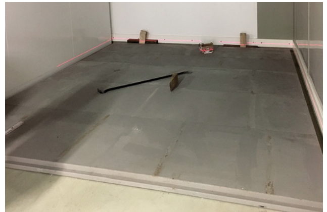
Installation of the vault floor
